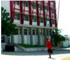
Faculty of Engineering and Computing
